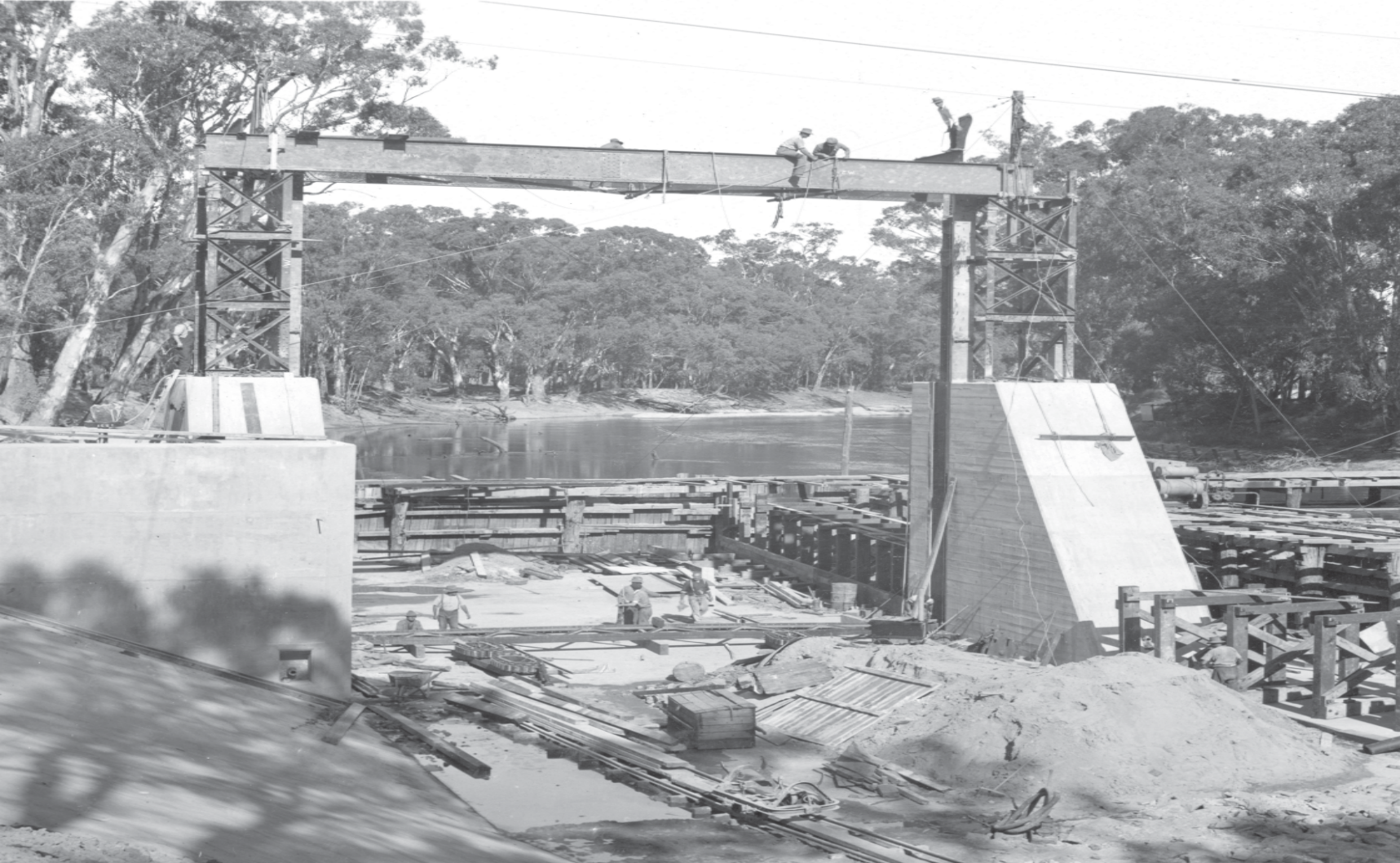
Under construction: Stevens Weir was built on the Edward River west of Deniliquin during the 1930s to provide water to the Wakool region. Photo: State Water Archive Collection
